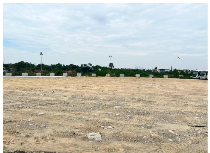
Photo 6: General view of the site
